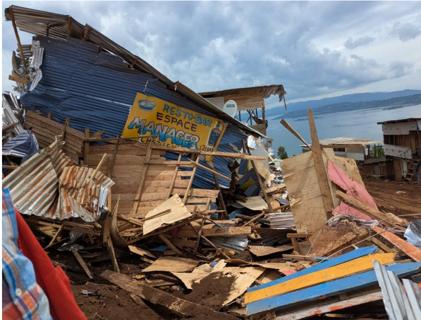
Structures belonging to civilians destroyed by M23 in April 2026 at the Lomera mining site in South Kivu province in the Democratic Republic of Congo. © Private
